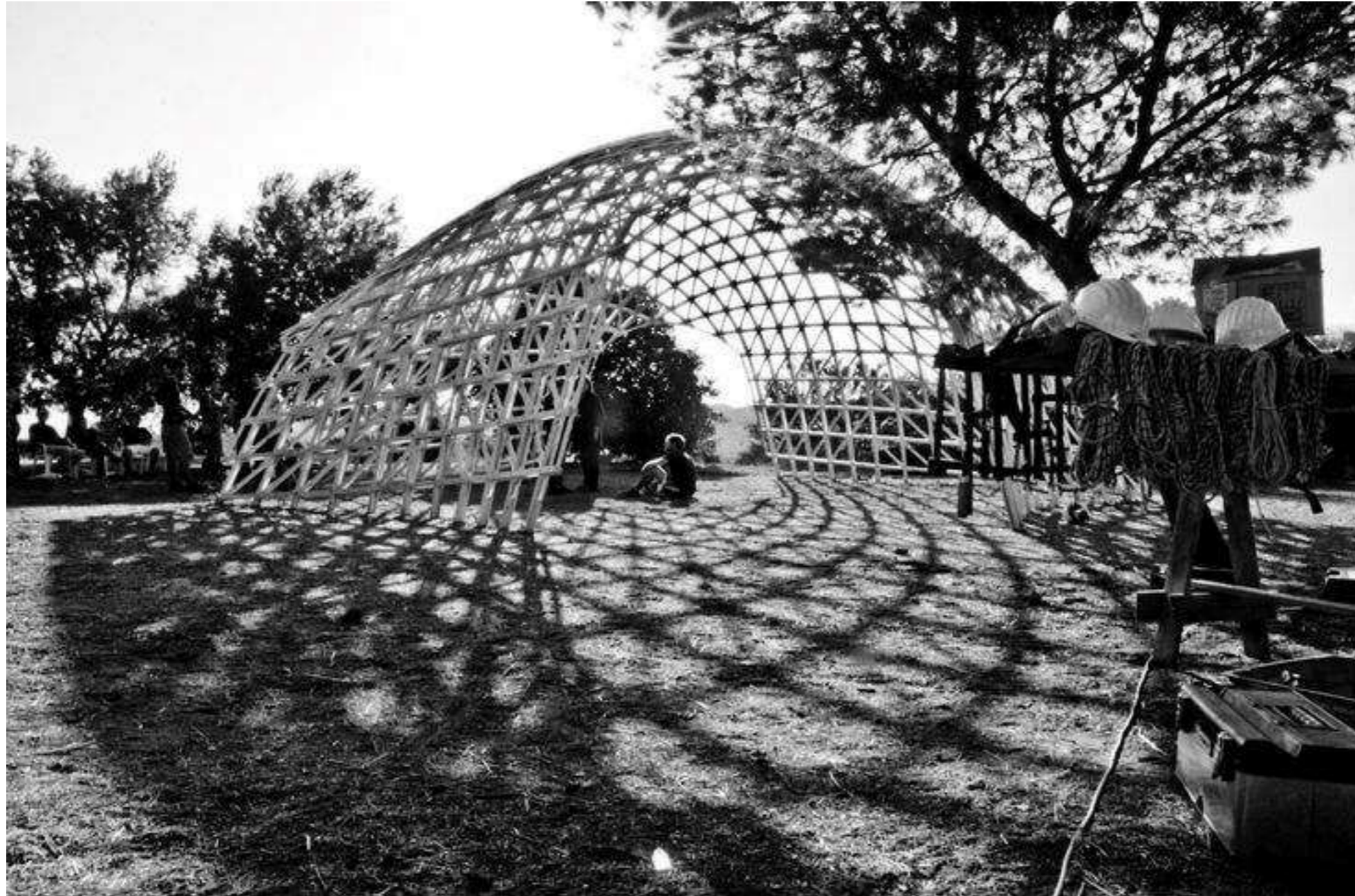
Gridshell Pavillion in the Archeological Park of SELINUNTE - lightweight form resistant wooden structures Source: www.gridshell.it
