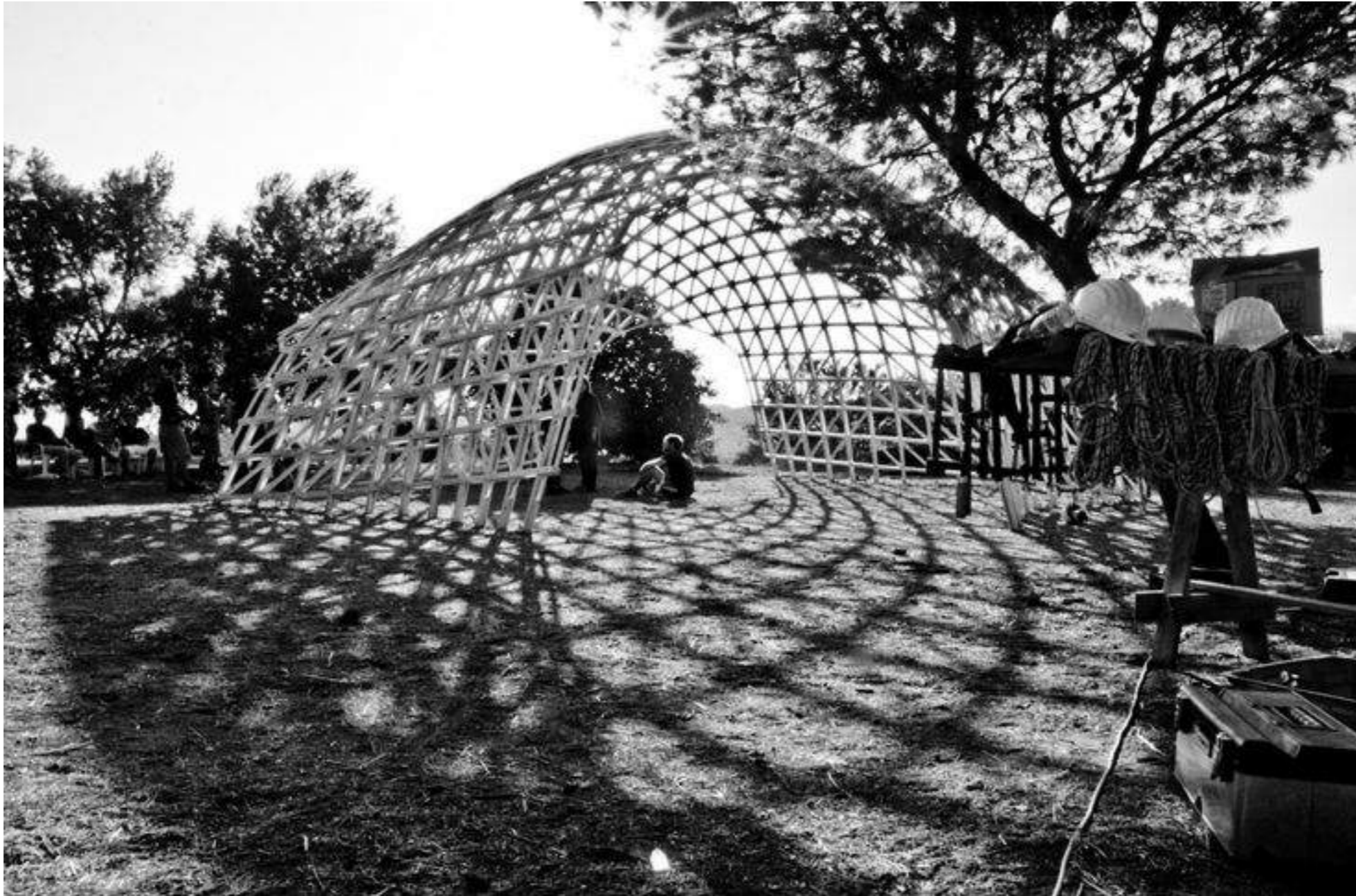
Gridshell Pavillion in the Archeological Park of SELINUNTE - lightweight form resistant wooden structures Source: www.gridshell.it
